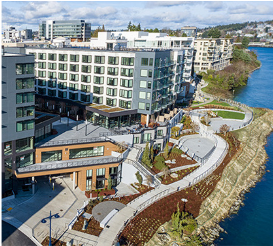
Marina Square Waterfront Apartments | Seattle, WA
