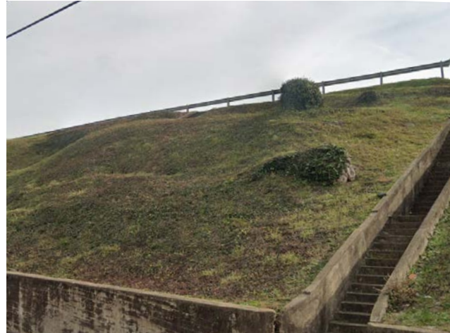
3. Existing Concrete Stairs along Sevier Ave.
